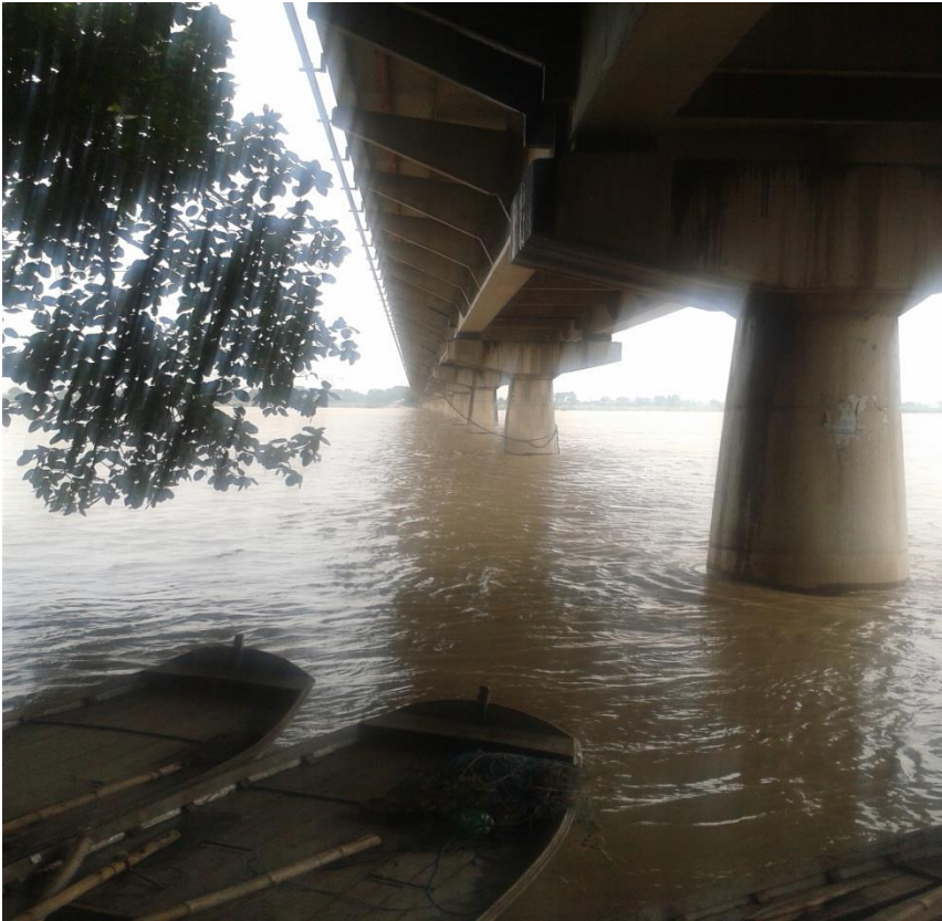
ANCHOR OF CAGE TO BRIDGE
