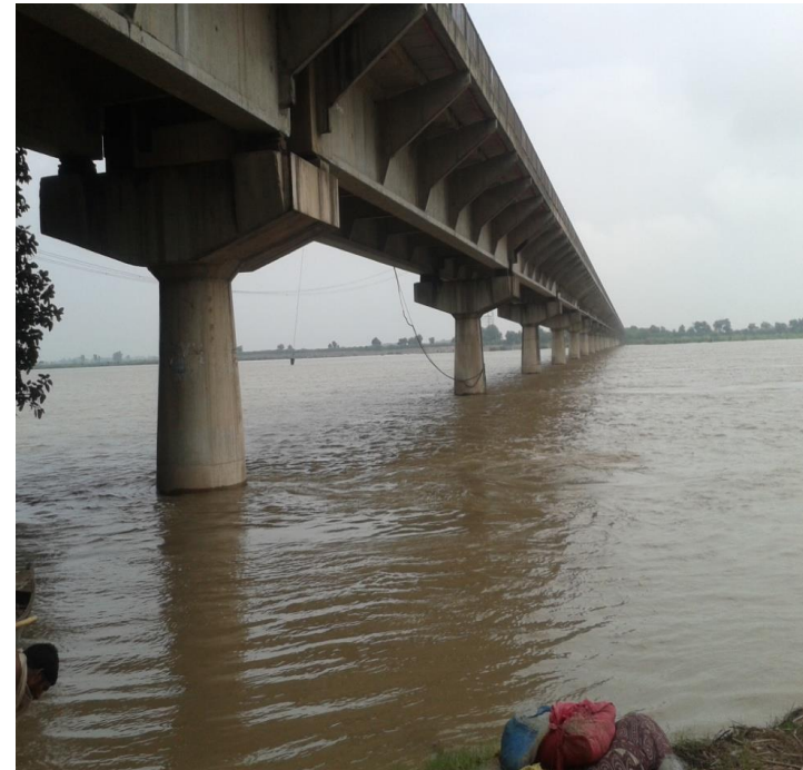
ANCHOR OF CAGE TO BRIDGE PILLAR
